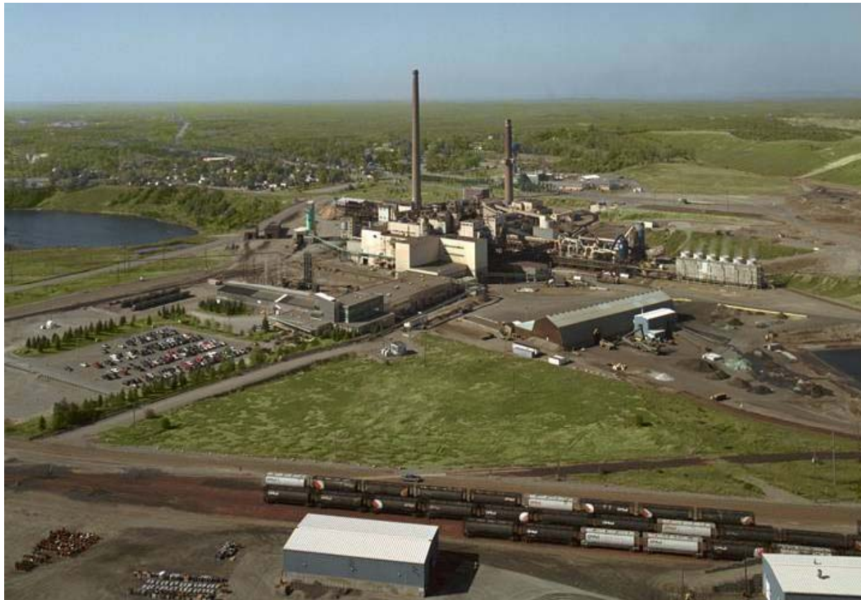
Aerial view of Xstrata Nickel Sudbury Smelter Falconbridge, Ontario, Canada
